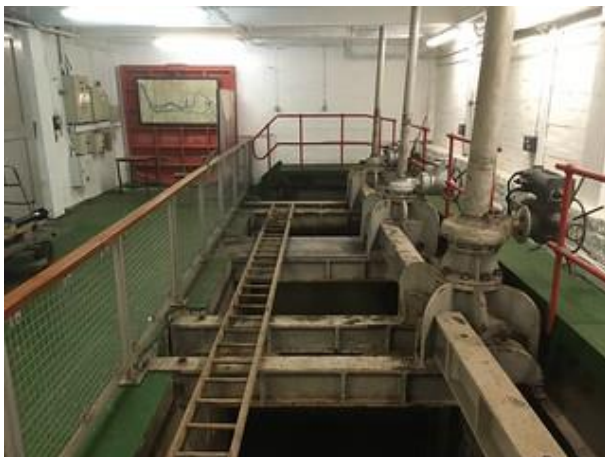
The Sluice Room illustrating the Tanks and Actuators
